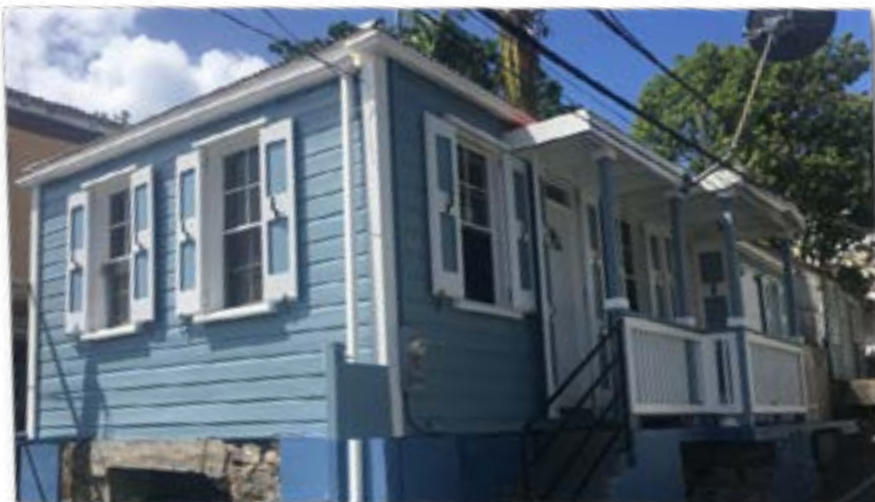
A Savanne rejuvenation project on St. Thomas, USVI, completed right after the impact of Hurricanes Irma & Maria on the Territory. - Photo submitted by the Enterprise Zone Commission.
