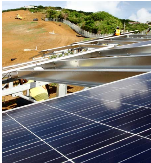
Estate Donoe Solar Project on St. Thomas
