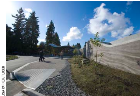
Rammed earth is a natural construction process that uses local materials such as earth, chalk, shells, and gravel. This is a historic process that has been brought back into use by the focus on sustainable building practices. Rammed-earth construction can be used for a variety of building types and purposes.
