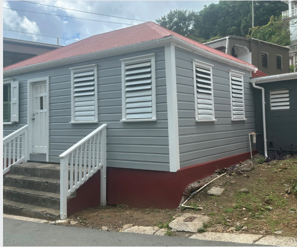
Alternate view of the EZC-supported restoration of a 100+ year-old building damaged in the 2017 storms (also featured on page 40).
