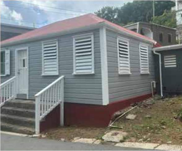
Alternate view of the EZC-supported restoration of a 100+ year-old building damaged in the 2017 storms (also featured on page 40).
